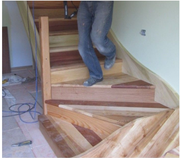
Jim McKeen making the staircase
