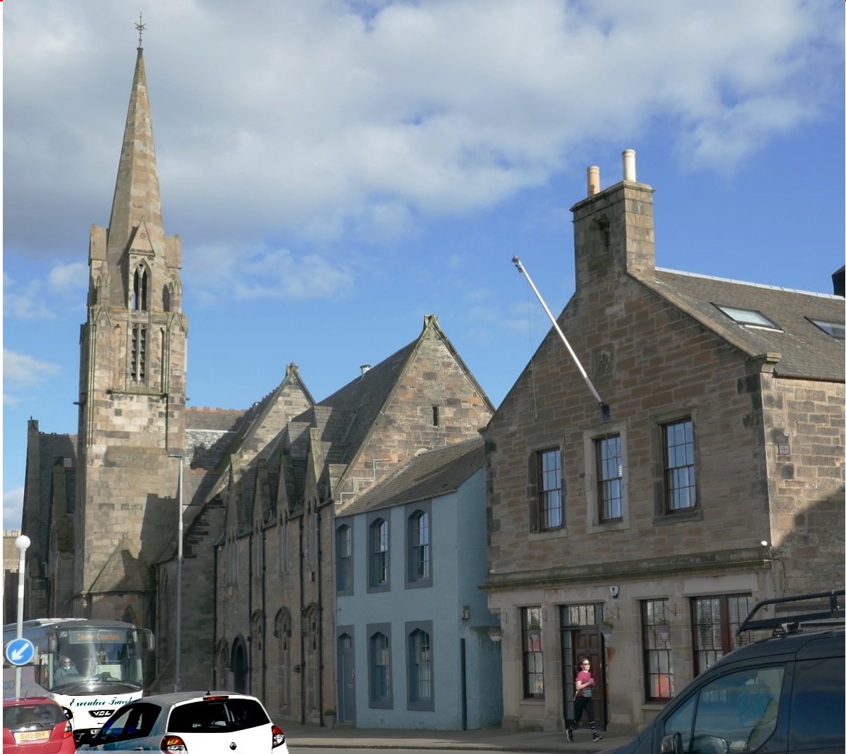
Old Newhaven Free Church with its accompanying halls, a fine group of buildings: the elegant spire has little gables rising higher than the corner pinnacles.
