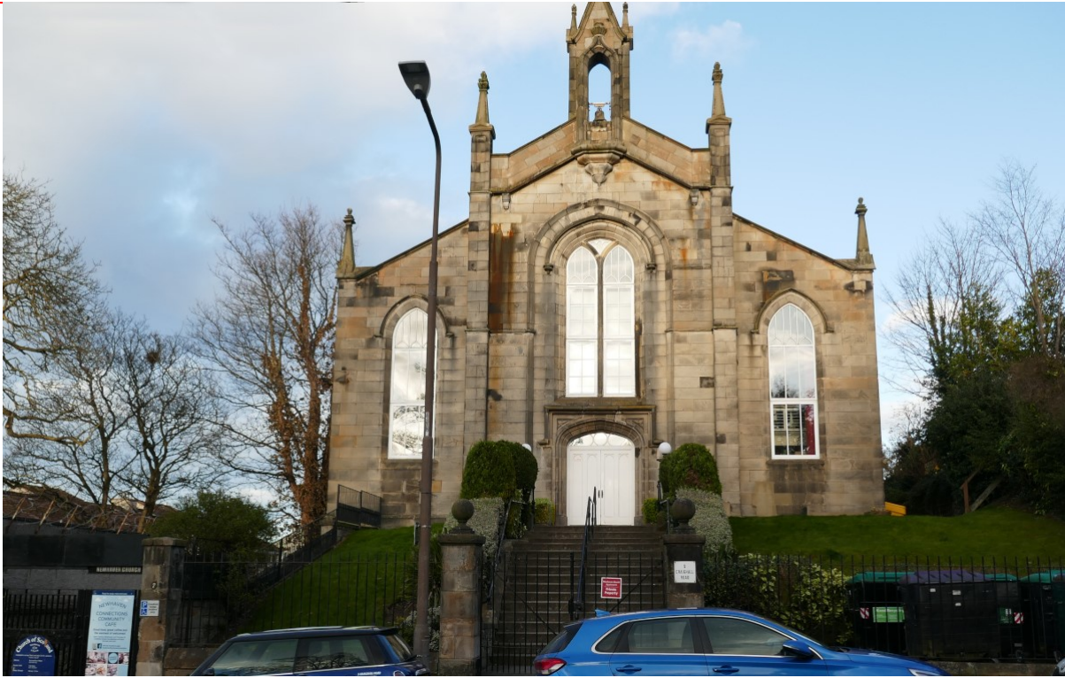
The west front of the former Newhaven Parish Church
