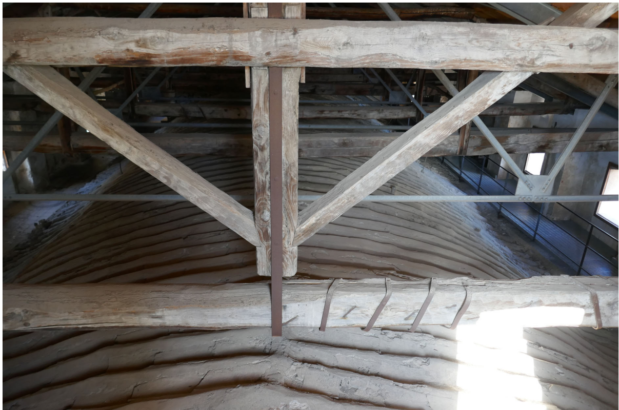
In the roof space, looking down on the vault, which seems to be constructed of tiles
