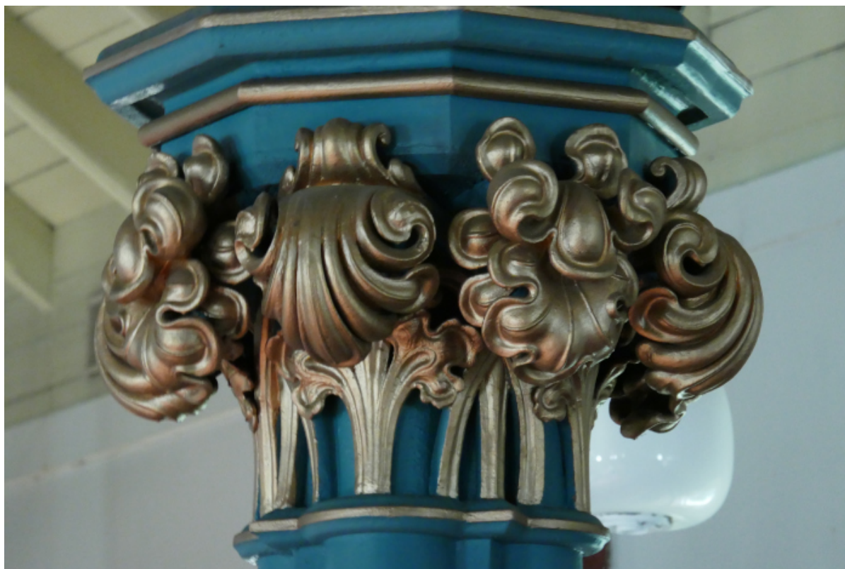
One of the sumptuous capitals of the cast-iron arcading which supports the galleries and the ceiling
